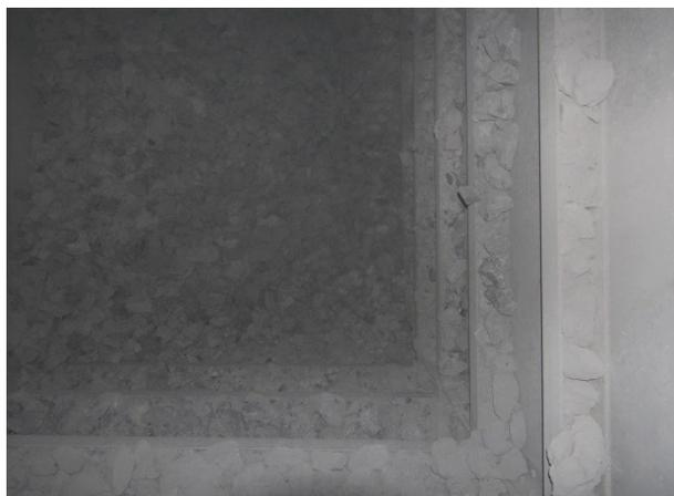
**Figure 2 Not an unusual view down inside a screen house bin with the typical design of reinforcing bars, creating ridges and product build up, which cause false signals to ultrasonic level sensors**
