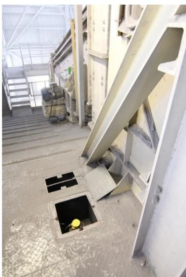
Figure 4: Sensors installed in the floor close to the screen infeed, but unaffected by in flight product and build up on the walls
