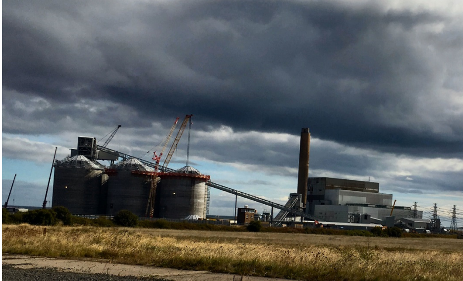
New Biomass Handling System Under Construction
