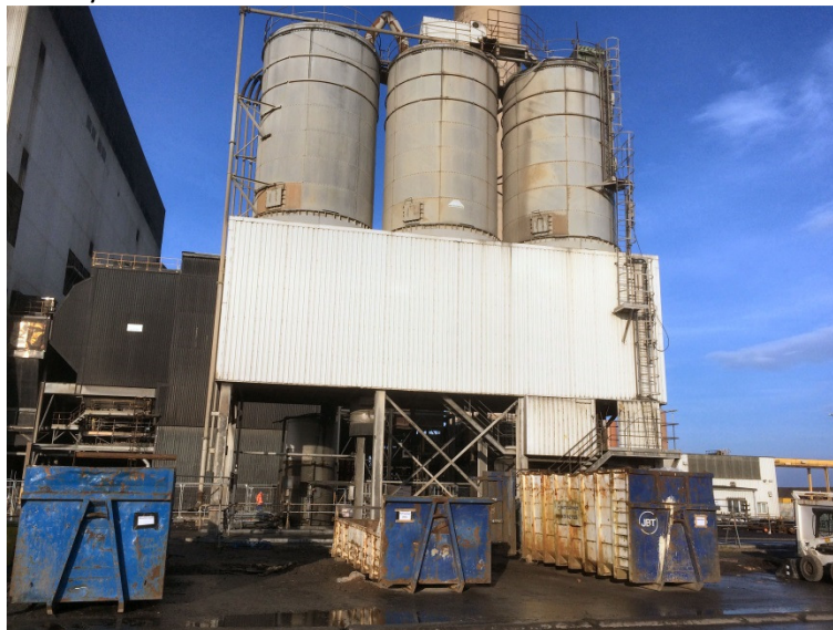
Existing Ash Disposal Facilities
