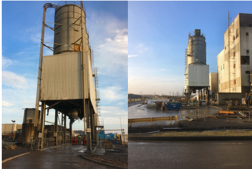
Existing Ash Disposal Facilities
