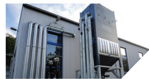
Explosion venting, one of the most common and effective forms of explosion protection, offers overpressure protection from potential industrial explosion hazards by providing a planned pathway for expanding gases and flame to escape.
