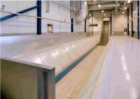
The Spiro Conveyor Floor employs a threecylinder hydraulically-driven aluminium floor profile system to convey loads with equal effectiveness in both of the following applications:
