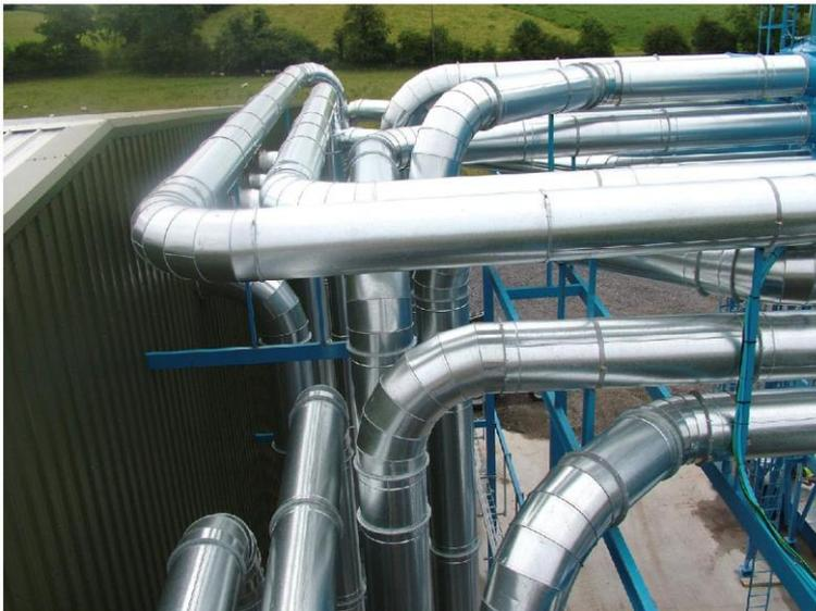
Careful design, with slow bends in place of tight ones, illustrated here with seven segments, and smooth aerodynamic branches and transitions will reduce fan power requirements – continuously. Incorrect air velocity in ducting can be expensive, not only in energy costs but also in maintenance and replacement costs. If it is too high, then fan power requirement can increase markedly; but also the rate of attrition will increase. This
