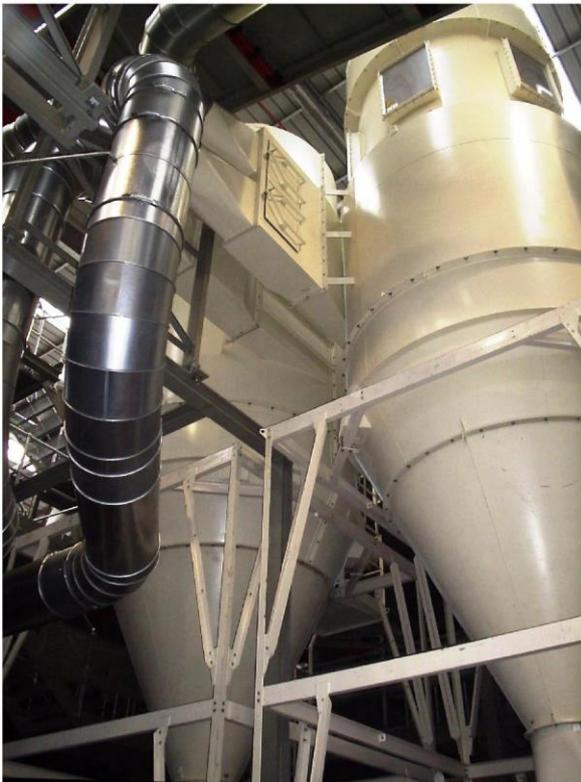
For example, cyclonic filters as illustrated occupy very little floor space, have a large dust capacity, but may be rather tall. Of course, there is a natural tendency to buy the smallest filter unit possible, to save space and initial cost. However, during its lifetime, the energy consumed by the extraction fan alone will probably cost more than ten times the capital cost of the entire installation. So, even small energy savings are well worth having and should be planned into the whole scheme.
