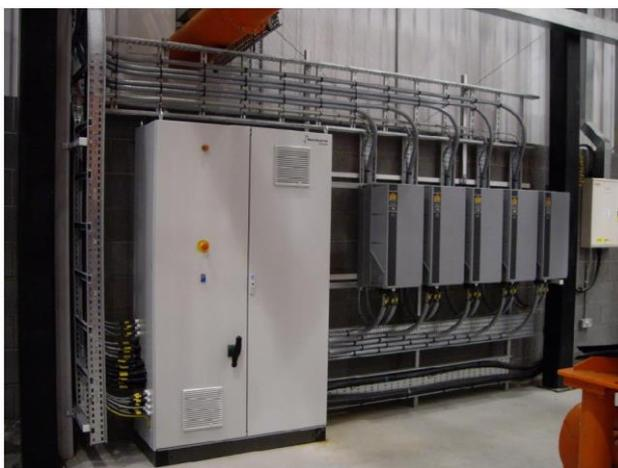
**Continuous modulation of the fan speed using an inverter drive could easily save in excess of £3000 every year in this example, without even taking into account the power losses of 5% or more incurred by belt drives.**
